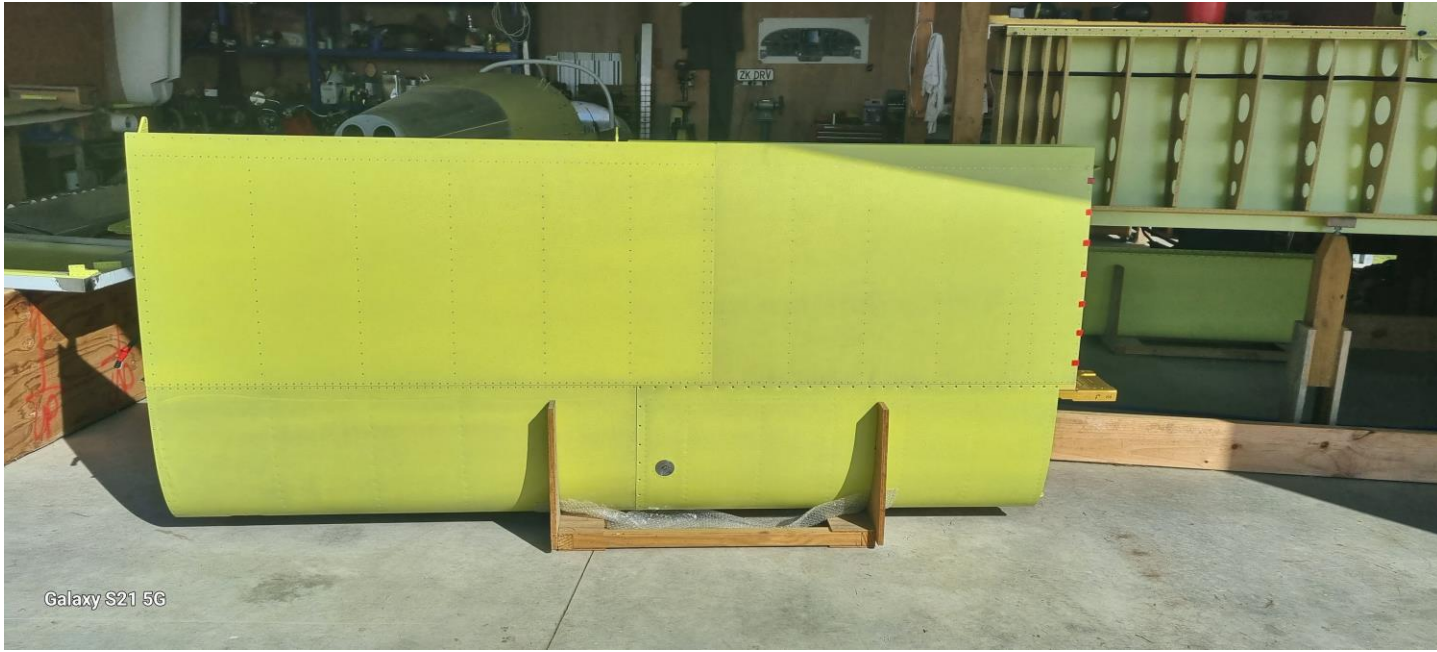
Above: Wing skins fully riveted on RH wing, and LH wing in background to right.
