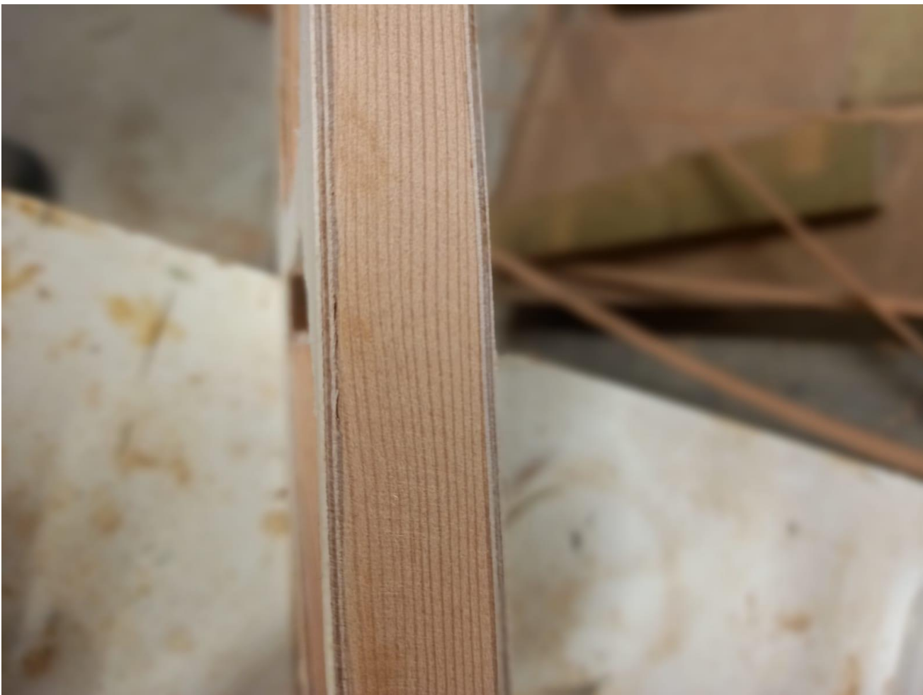
Photo showing birch ply either side of Oregon in ribs...
