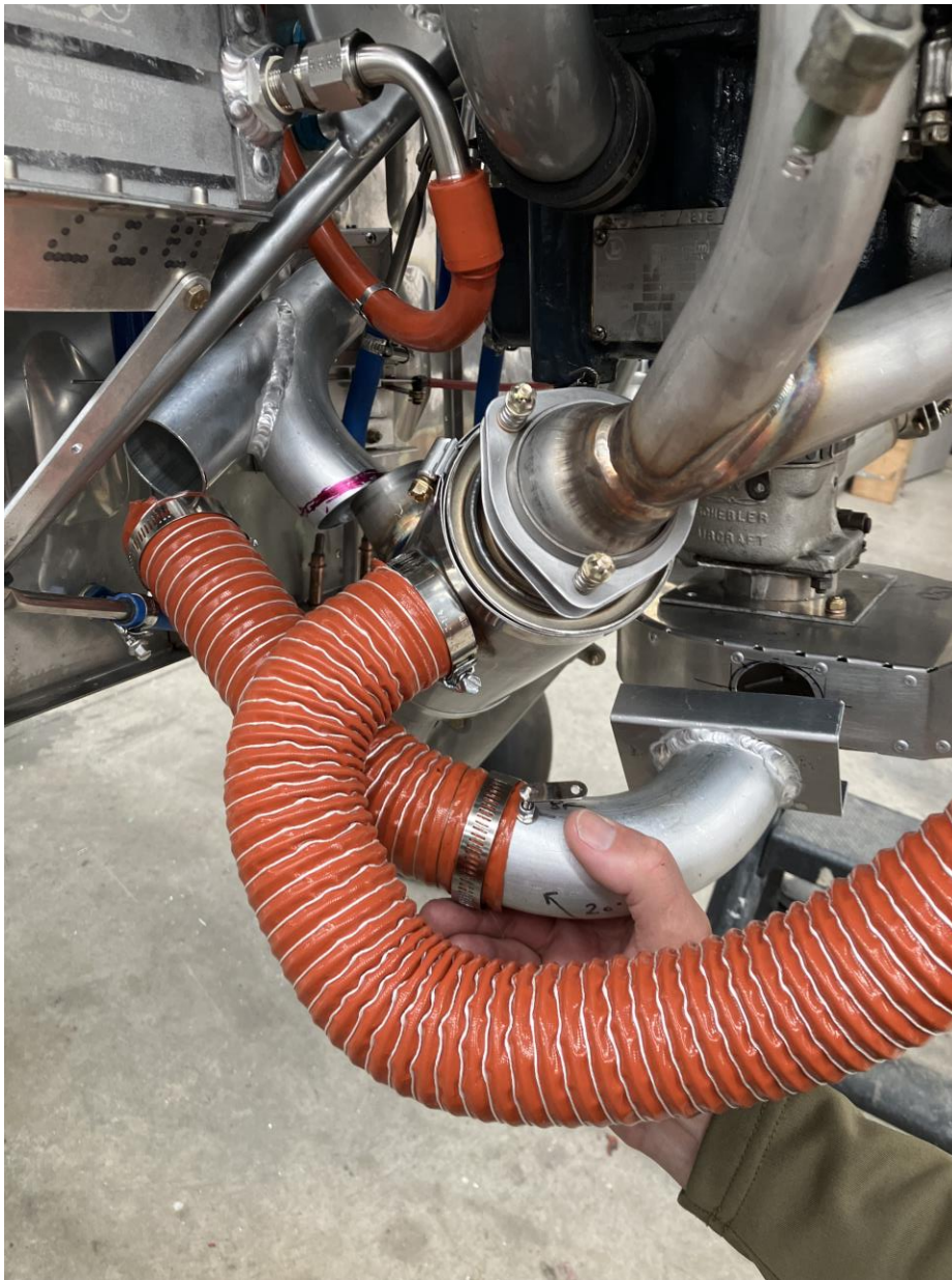
Above: Carb Heat box fitting up hot air ducts
