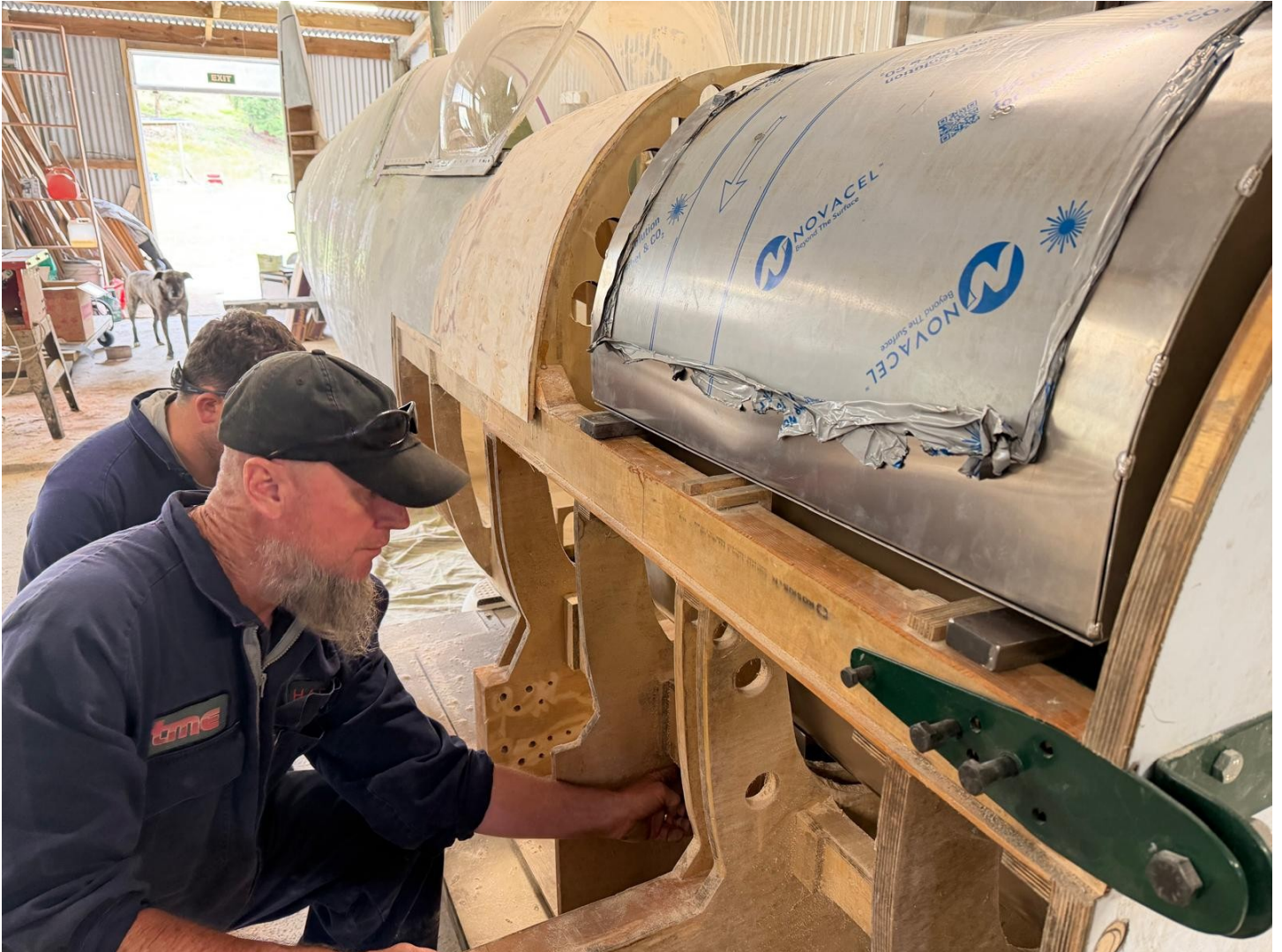
Below: Fitting Tank, view from other side
